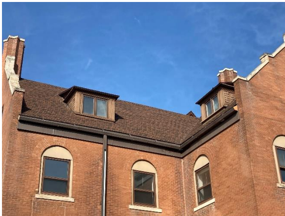
Temporary Asphalt Roof @ Babcock
