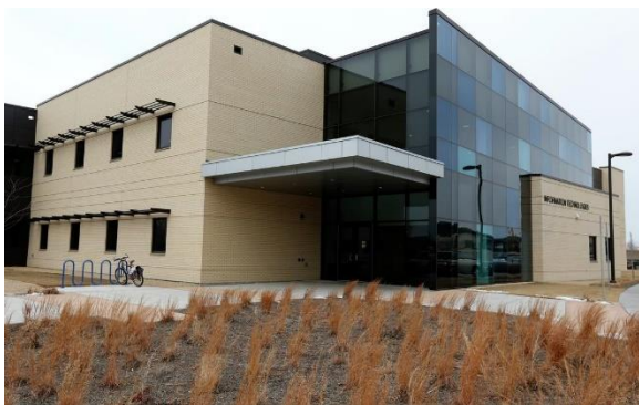
Main Entry IT Building
