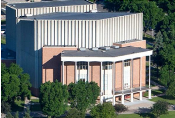
Pre-Cast Wall Panels @ The Fritz
