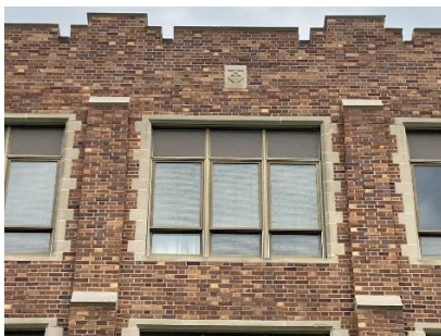
Stone Quoining at Windows
