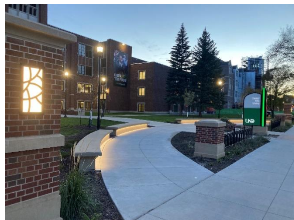
Task Lighting beneath seating and within masonry column
