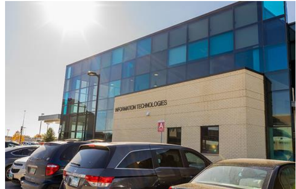
West Facade of Information Technology
