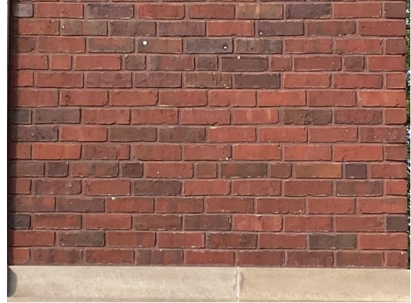
Carnegie Brick Restoration with matching mortar color
