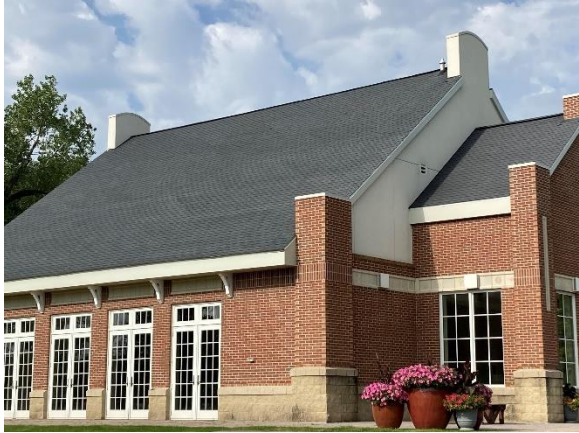
Asphalt Roof @ Hopper Danley Chapel
