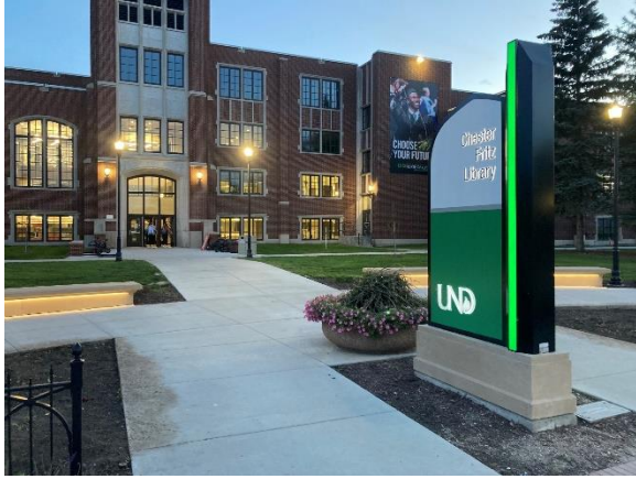
Ambient Lighting at post and wall sconce
