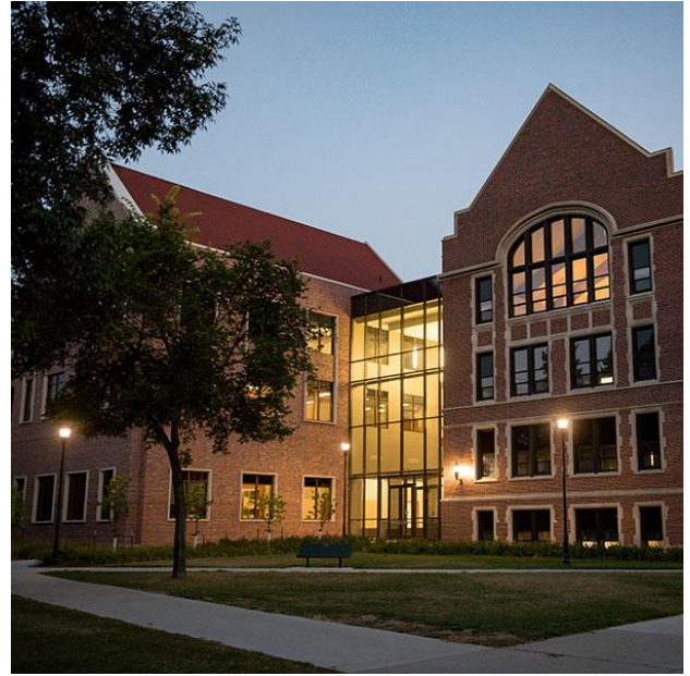
School of Law Addition Transitional Contextual; Original Building Traditional
