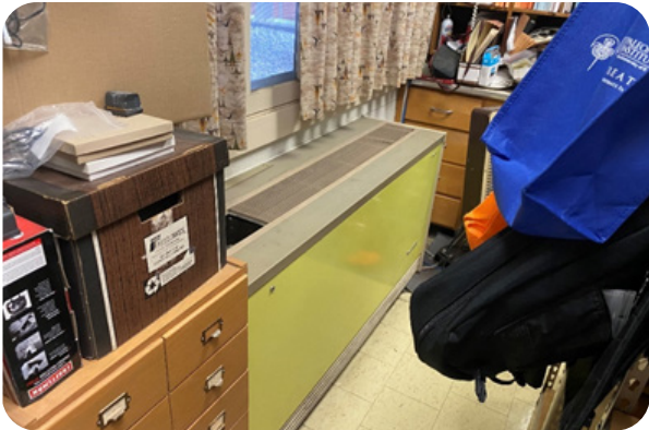
FIGURE 4.12 Typical Unit Ventilator
