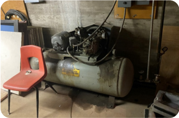
FIGURE 1.2 Controls Air Compressor
