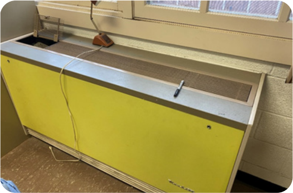
FIGURE 4.13 Typical Unit Ventilator
