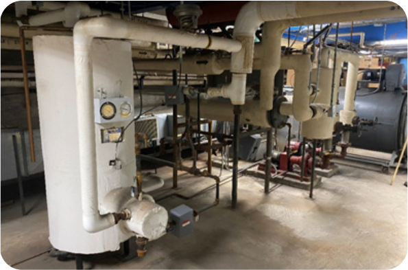
FIGURE 3.1 Domestic Hot Water Generator, Steam Heat Exchanger, Heating Water Pumps
