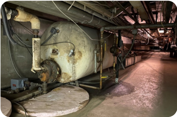
FIGURE 1.4 Domestic Water Heater
