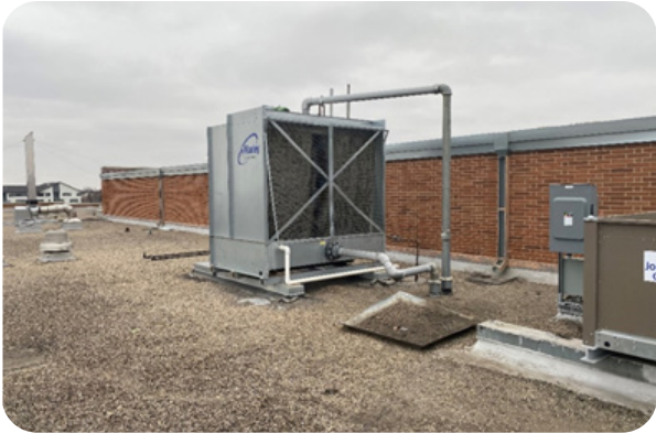
FIGURE 4.8 Fluid Cooler
