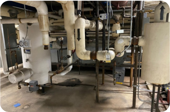
FIGURE 3.3 Steam / Heating Water Heat Exchanger
