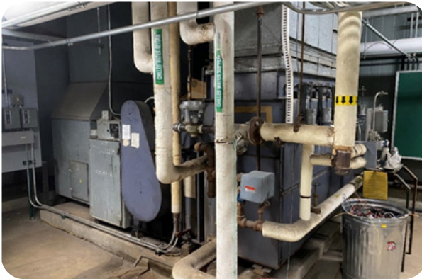
FIGURE 1.10 Steam Pressure Reducing Station
