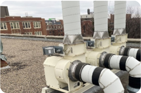
FIGURE 1.17 Lab 321 Hood Exhaust Fans
