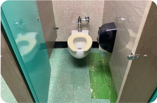
FIGURE 4.14 Typical Wall Hung Water Closet
