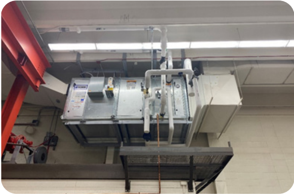
FIGURE 3.26 Air Handling Unit AHU-1
