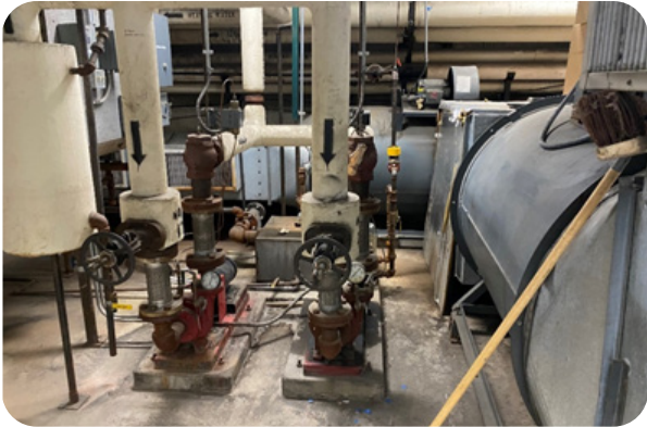
FIGURE 3.2 Heating Pumps
