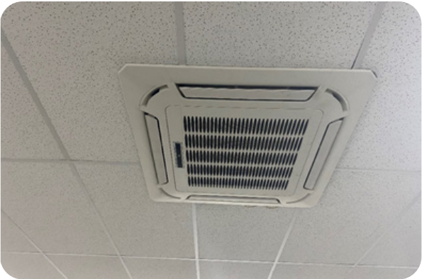
FIGURE 4.11 Typical Ceiling Mounted Mini-Split Cooling Cassette
