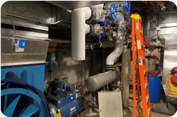
FIGURE 3.10 Steam Heat Exchanger
