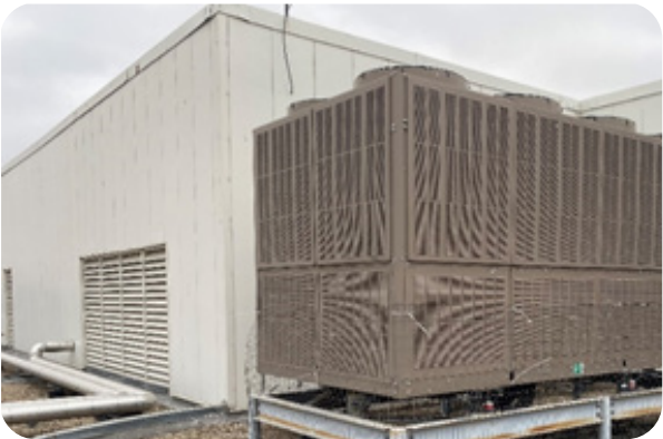
FIGURE 1.15 New Chiller (2014) for Lab 160 MAU AHU-13
