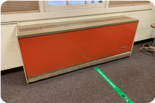
FIGURE 4.10 Typical Unit Ventilators
