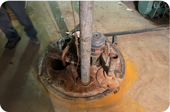
FIGURE 1.3 Sewage Ejector Pump
