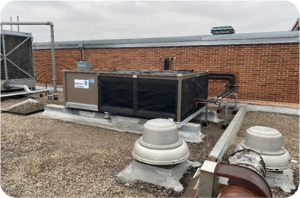
FIGURE 4.7 Air Cooled Condensing Unit
