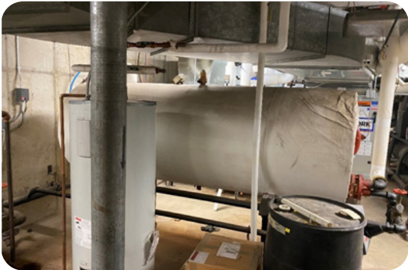
FIGURE 4.6 Domestic Water Generator
