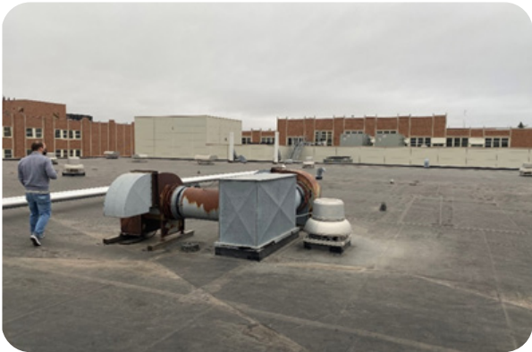
FIGURE 3.22 Welding and Wood Shop Exhaust Fans
