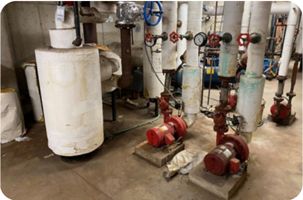
FIGURE 4.5 Heat Water Pumps
