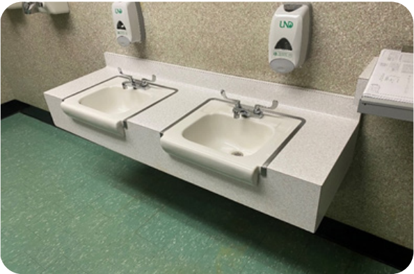
FIGURE 4.15 Typical Wall Hung Lavatories
