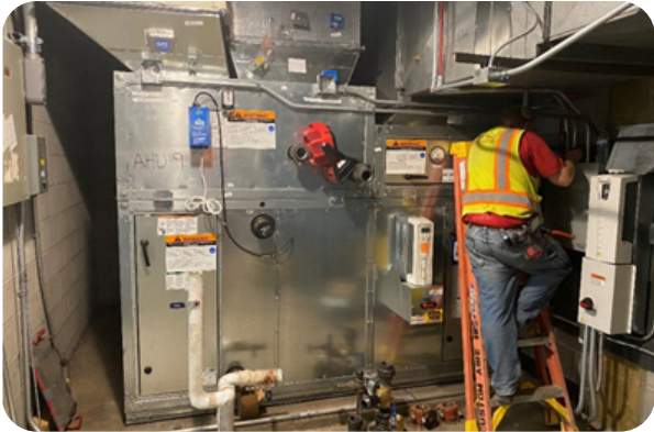
FIGURE 3.8 Air Handler AHU-9
