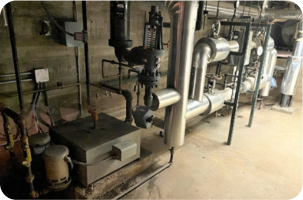
FIGURE 1.1 Steam Pressure Reducing Station
