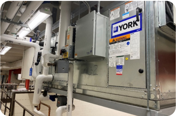
FIGURE 3.29 Air Handler AHU-2
