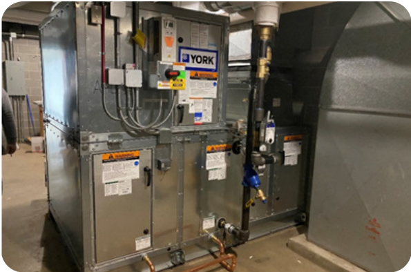
FIGURE 3.6 Air Handler AHU-10
