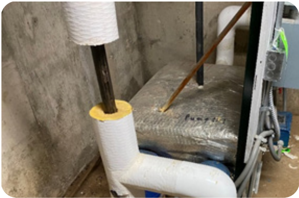
FIGURE 2.4 Condensate Pump
