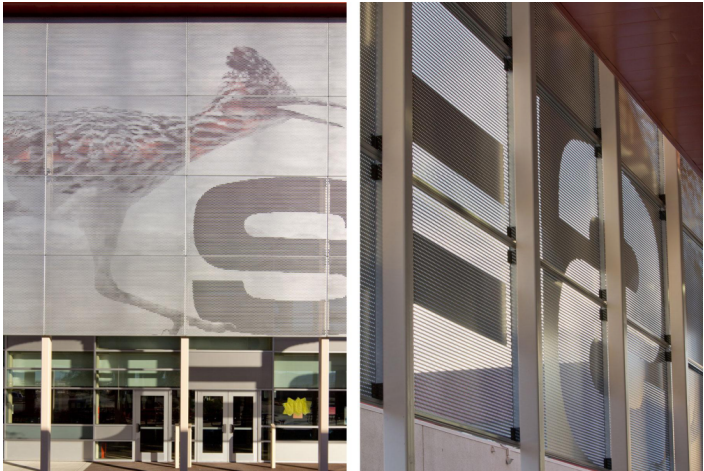
PERFORATED METAL PANEL SCREEN SYSTEM
