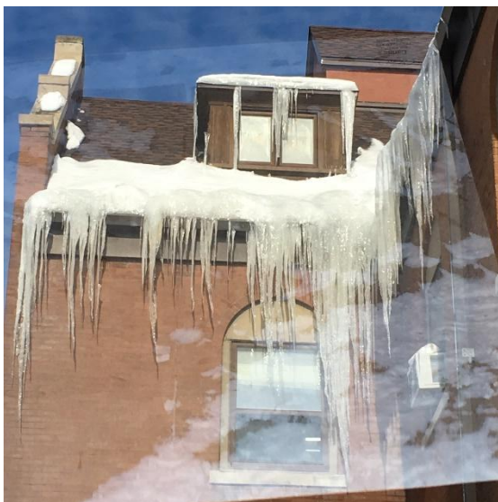
Babcock Roof Lack of Insulation & Venting
