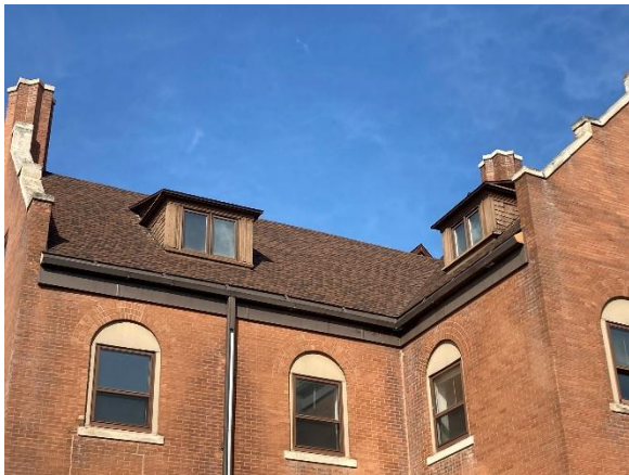
Temporary Asphalt Roof @ Babcock
